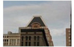
Deutsche Bank building with missing capstone, New York City
